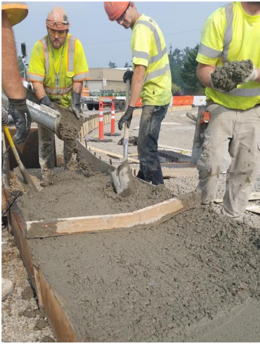
Building a rolled curb for emergency vehicles and trucks
