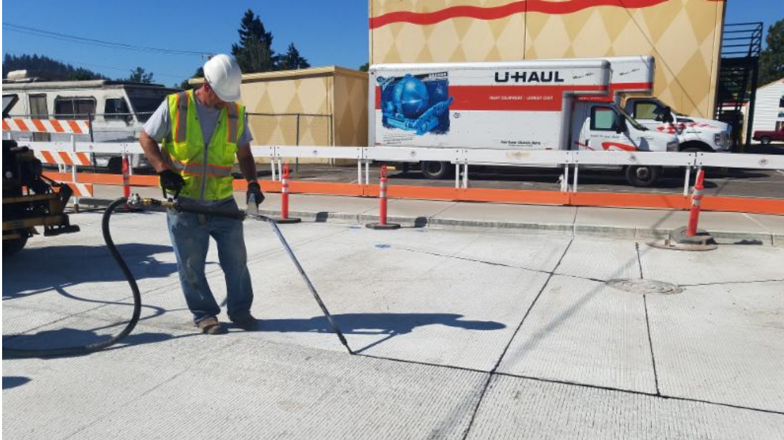
Sealing the joints ensures the longevity of the new road
