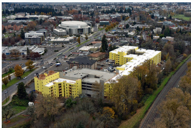
Transit-oriented development is already responding to Franklin Boulevard's BRT line, causing a need to expand capacity and upgrade the streetscape. This photo shows the Matthew Knight Arena in the background, new housing, and hospitality development in the foreground built around the EmX Walnut Station.
