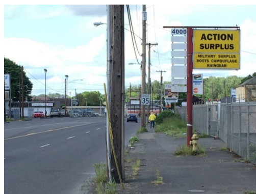
Sidewalk gaps, a lack of bike facilities, and degrading pavement condition will all be remedied, upgrading Franklin to a state of good repair.
